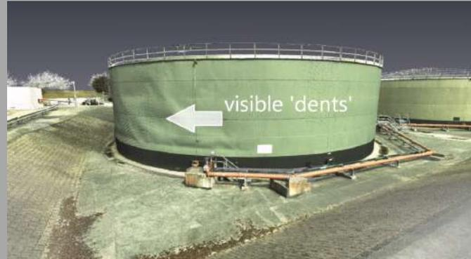
Dents visible in the tank shell needed to be quantified
